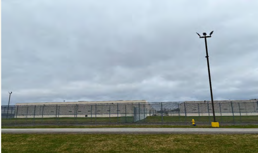
Moshannon's no-climb fence upgraded for ICE
