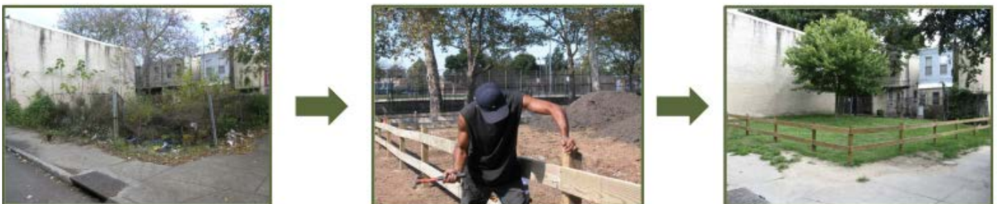
Figure 2. Process of transforming a vacant lot.
